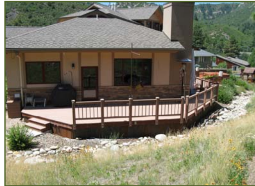
Kurz installed rusted corrugated steel under his deck and steps to prevent the accumulation of debris and/or flying embers from becoming lodged underneath.
