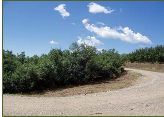
Line of sight was improved at many of the curves along the subdivision's roads.
