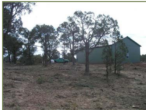
Back side of the fire station after mitigation.
