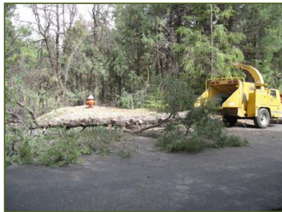
Clearing around a fire hydrant to make it more visible and accessible.
