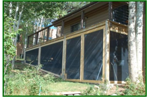
The FireWise Ambassador had the area beneath her deck screened in to protect the area from flying embers.
