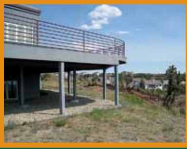
Figure 14: This homeowner worked hard to create a defensible space around the home. Notice that all fuel has been removed within the first 5 feet of the home, which survived the Waldo Canyon Fire in the summer of 2012. Photo: Christina Randall, Colorado Springs Fire Department
