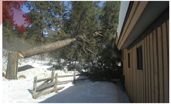
Too close to structure.
