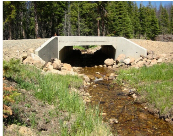
Typical AOP designs for road crossing. Photo source: https://www.greatwesteng.com/aop/
